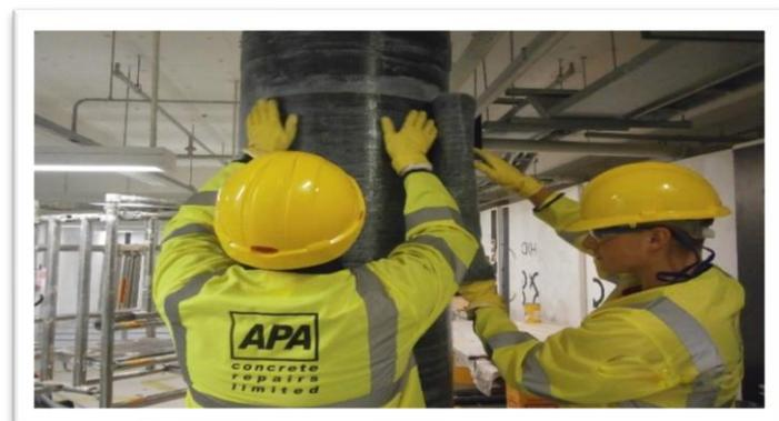
**The outcome:** The works allowed for much of the carpark to remain in active use throughout, thereby creating minimal disruption to the centre's everyday activity. Due to the carbon fibre composite strengthening completed by **APA**, the reinforced columns, complete with the added assurance of two hours fire resistance, provided the increased load carrying capacity to enable the additional floor level to be constructed.
